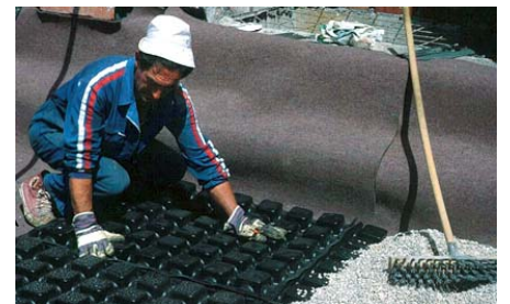
Installation of the Drainage Elements Floradrain® FD 60.
