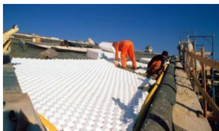
Installation of the drainage element Floraset® FS 75 on the pitched green roof area.
