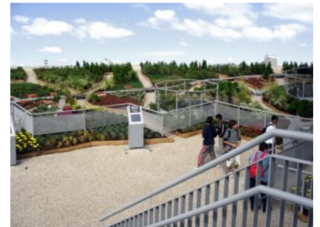
The stairs descend to an accessible area amidst the green roof.
