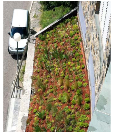
Despite the alpine mountains of Andorra, with their frequent rainfalls, the roof gardeners decided to install a drip irrigation.
