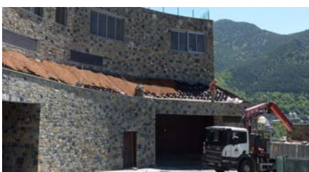
The difficulty for the roof gardeners was the professional handling of shear forces on this steep roof area.
