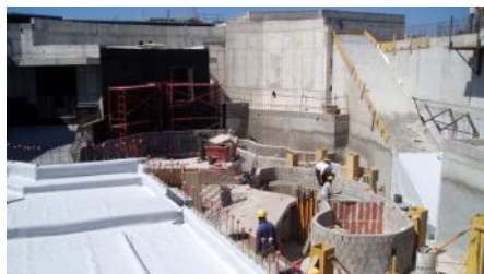
Installation of the root barrier WSB 80-PO.
