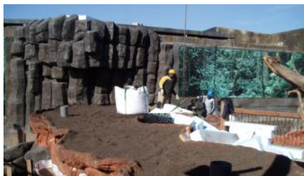
Delivery of substrate on top of the Filter Sheet SF.
