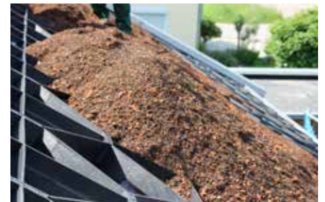
The system substrate “Heather with Lavender-light” is, e.g. delivered in a silo tanker. It is then blown onto the roof until the Georaster® elements are filled and covered up to about 10 mm over their upper edge.
